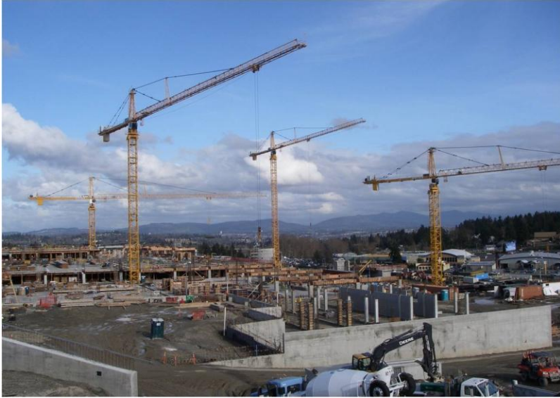
Project View from Bridge #4
