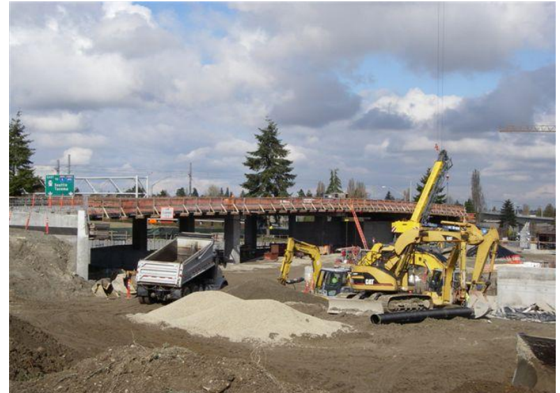
Bridge #4 Progress: Girders in Place
