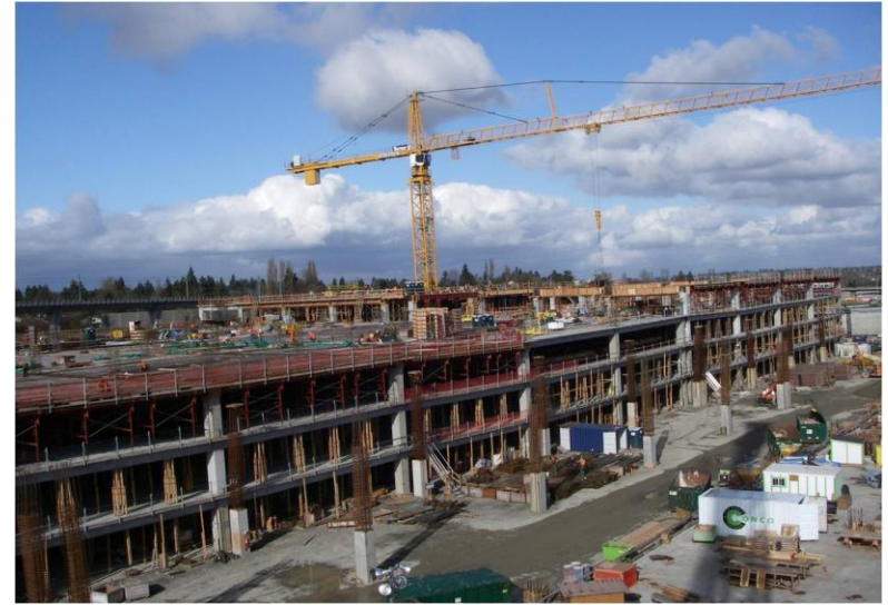
Elevated Decks in Areas A, B and C
