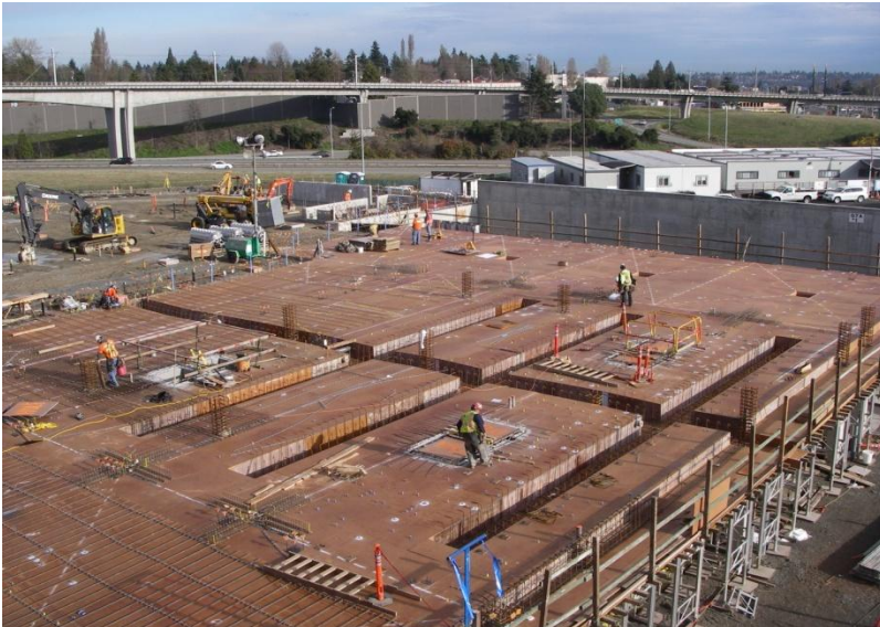
QTA #2: Elevated Deck Forms
